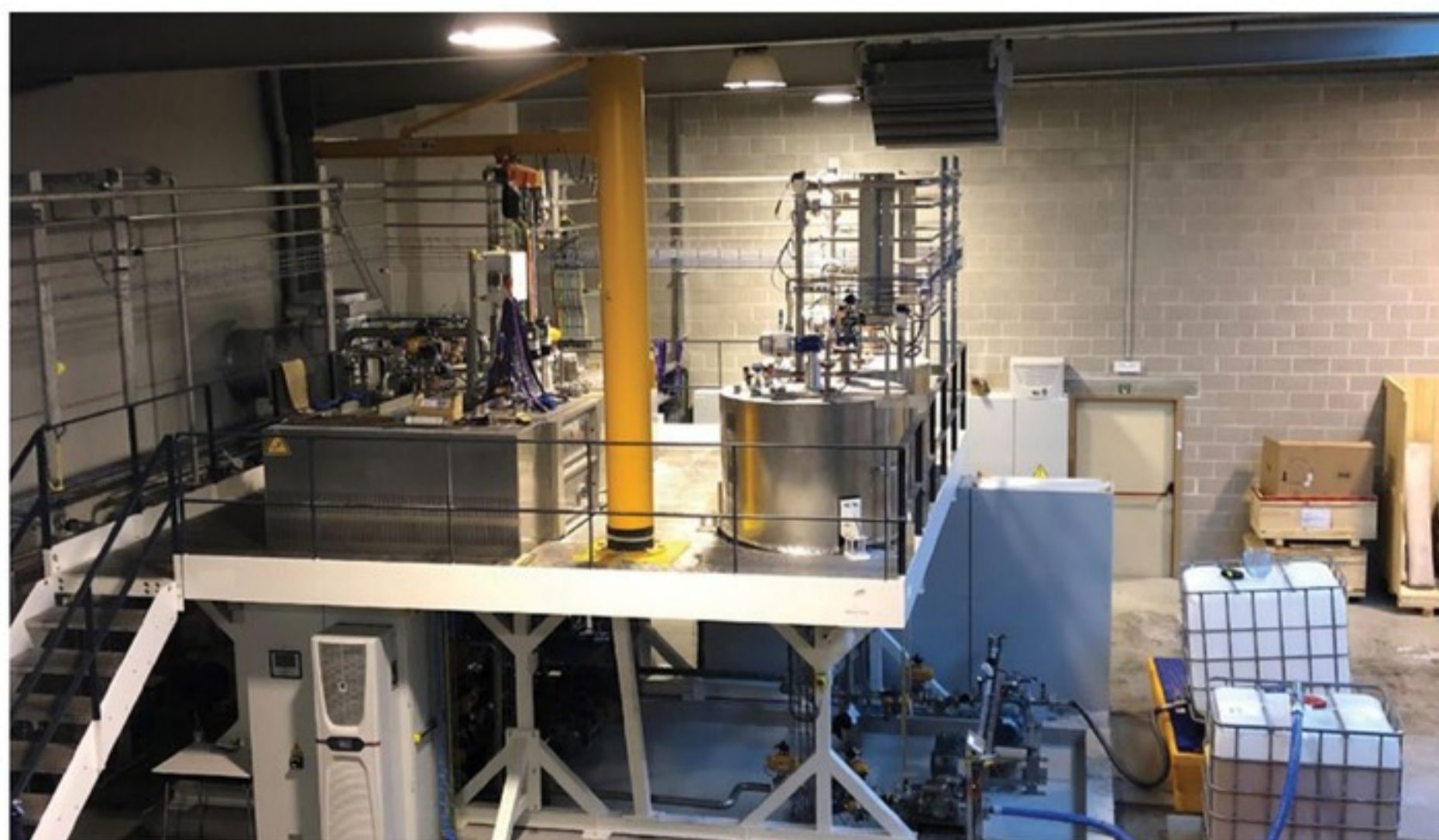
Processing equipment at Green Frix
